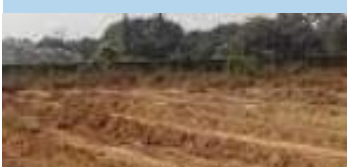
Site clearance, fencing etc
