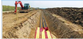
Cable installation earth works
